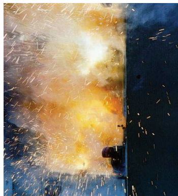
Photo courtesy of Schneider Electric
