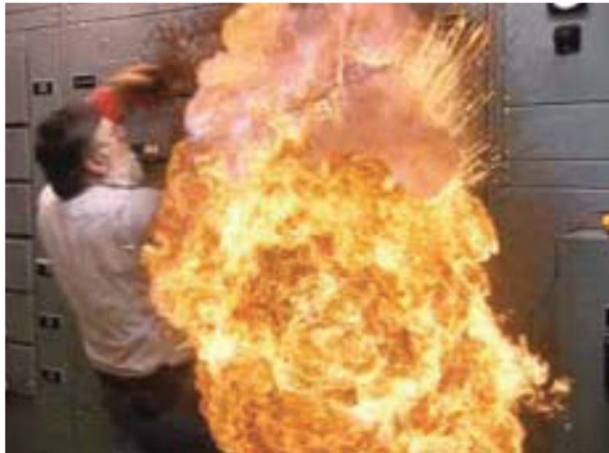
Photo of arc flash incident.
