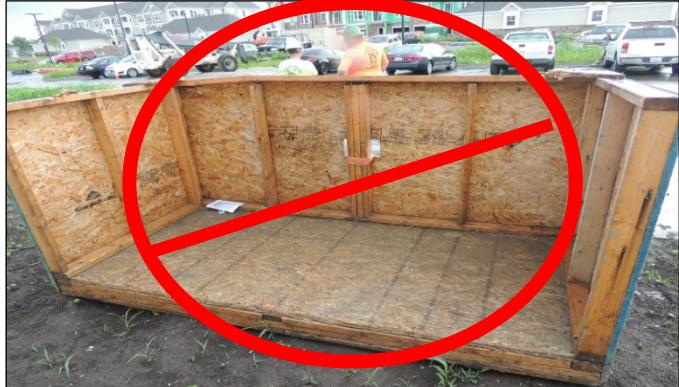
A typical job-made box consists of a wooden (e.g. plywood) platform with three walls. In this example, the job-made box was attached to a powered industrial truck (PIT) using a strap looped around the center of the wood beams that make up the longest wall and a galvanized hook. A worker was injured when the hook’s safety latch failed and the platform fell to the ground.
