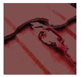
**Install an anchor above the area being built:** Choose an anchor that is appropriate for the tile type and anchor location. Depending on the roof
