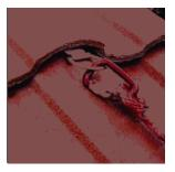
Install an anchor above the area being built: Choose an anchor that is appropriate for the tile type and anchor location. Depending on the roof design, the best location might be at the peak of the roof, directly over a truss.
