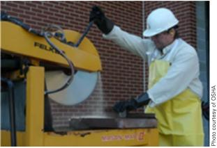
A worker cutting masonry block on a stationary masonry saw that continuously feeds water to the blade.
