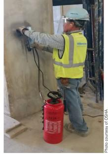
Example of a handheld grinder with integrated water delivery system.
