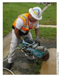
A construction worker using a handheld power saw with an integrated water delivery system.
