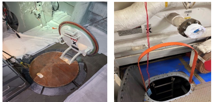
(Left) Image shows a hatch cover with adequate covering. (Right) Image shows appropriate use of a "U" bar to temporarily guard flush manholes during shipbuilding and ship repair operations.
