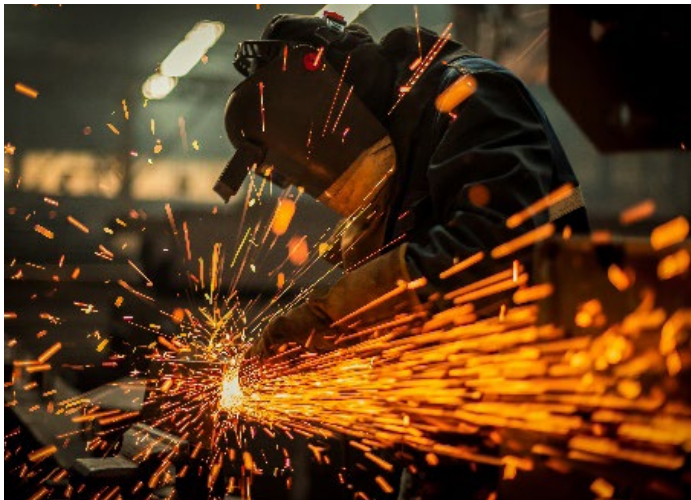
Figure 2: Welder performing hot work.
