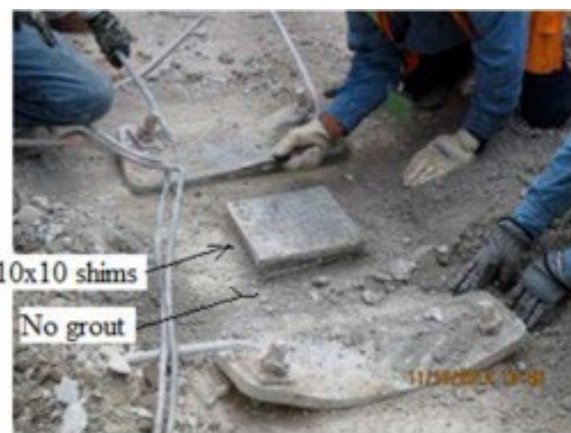
Figure 2: Column base plate and shims
