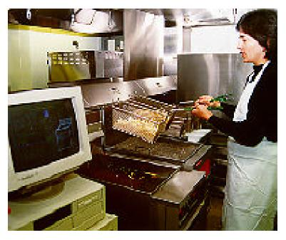
found even higher CO levels. This time, the maintenance worker re-adjusted the fryer flame and found that a fire damper in the hood air supply duct was closed. FINDINGS: Fryer generating excessive CO and exhaust hood no longer able to remove CO due to insufficient make-up air caused by closed fire damper. CO released into work area.
