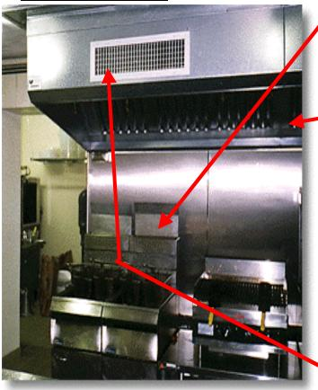
Many fryer units are portable and do not directly exhaust outdoors. Portable fryer units require an additional ventilation system to exhaust combustion gases outdoors.
