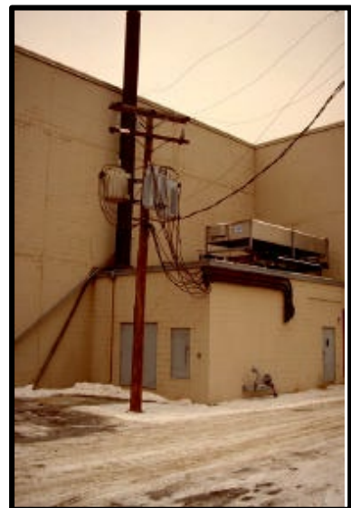
Service Drop Line
