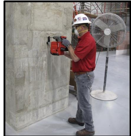
***Work performed indoors or in enclosed spaces requires a means of exhaust, such as a portable fan, to minimize the accumulation of visible airborne dust.***
