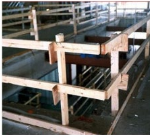
Properly installed guardrail system.
