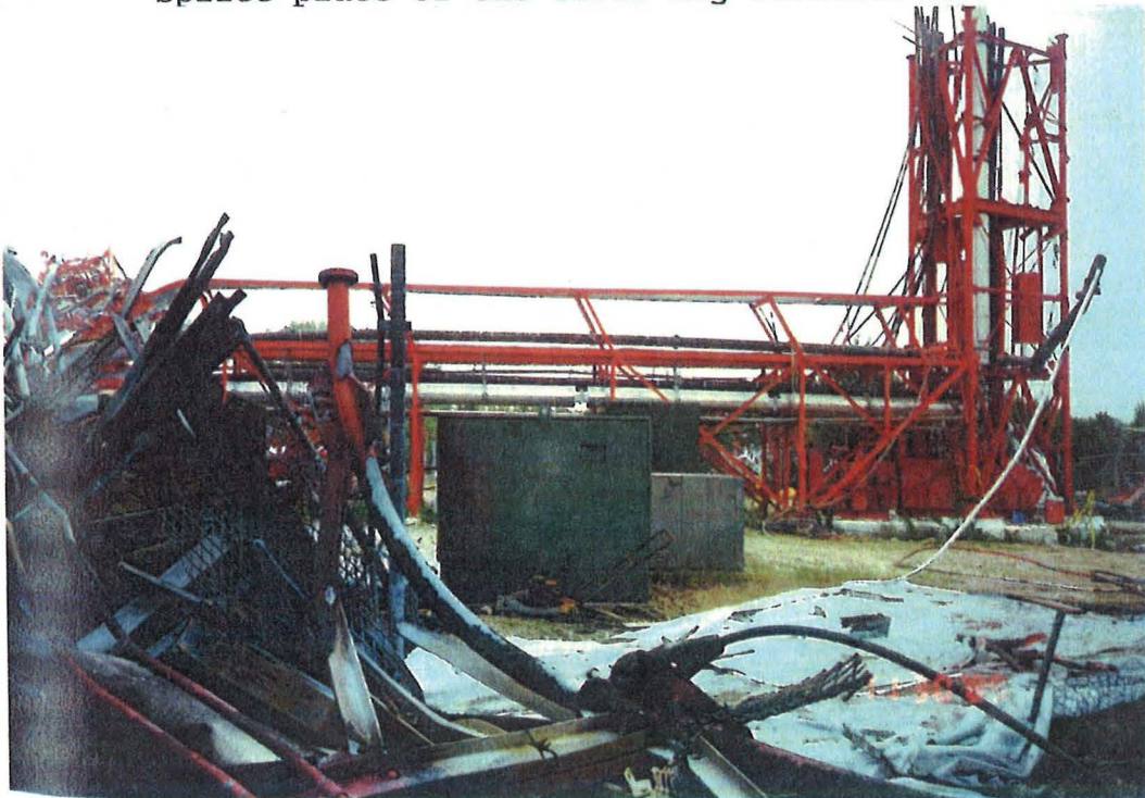
The bottom section (30' long) remained generally intact during the collapse.
