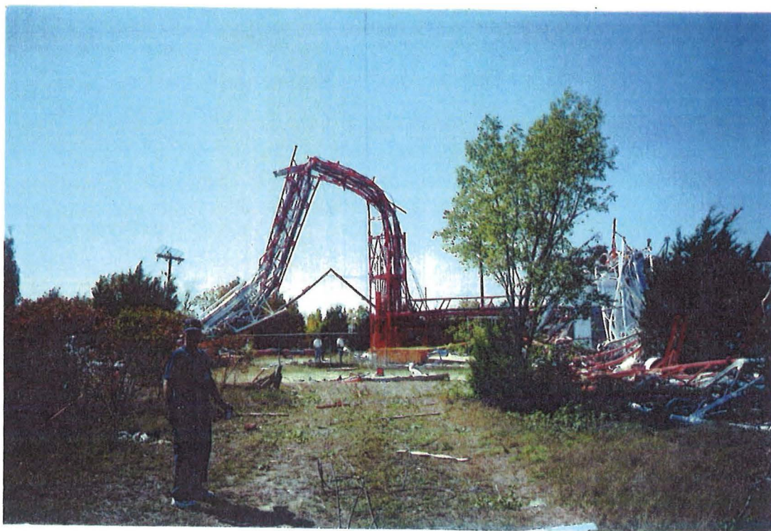
General View of the Collapsed Tower.
