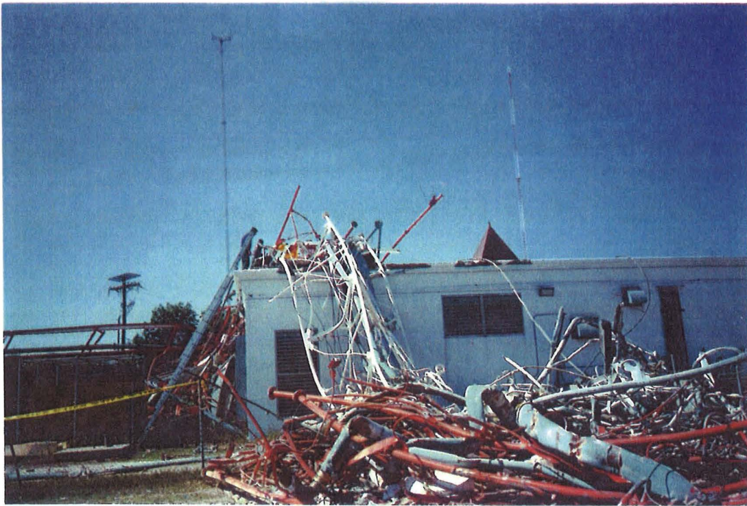
Scene of the collapsed tower. Part of the tower fell over the transmission building. Section #8 with the track attached to it was found on the roof.
