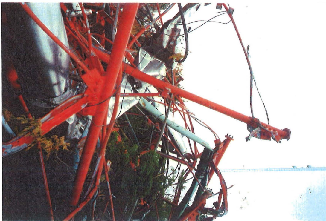
Views showing typical connection of the diagonal and horizontal struts to the tower legs.
