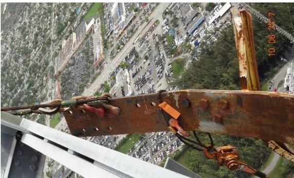
*Figure 26 – Close-up of Plastic Hinge in Top Track Plate (provided by Stainless)*
