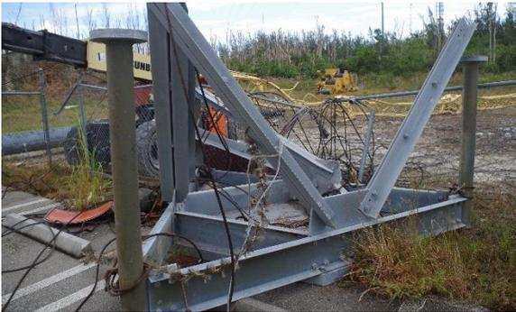
Figure 19 – Dummy Pole Pedestal
