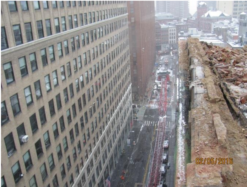
Figure 5 Boom and jib on the ground after the incident – aerial view.
