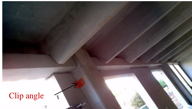
Fig. 33 Wall panel connected by clip angle to column (post-incident)
