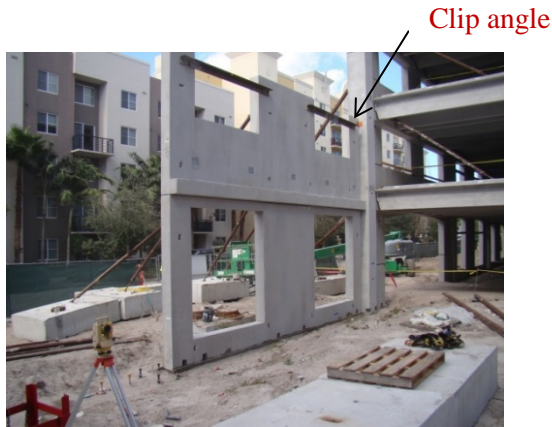
Fig. 32 Wall panel connected by clip angle to column (post-incident)
