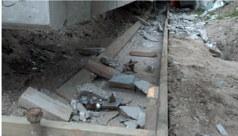
Fig. 14 Lumber as a formwork for the grout
