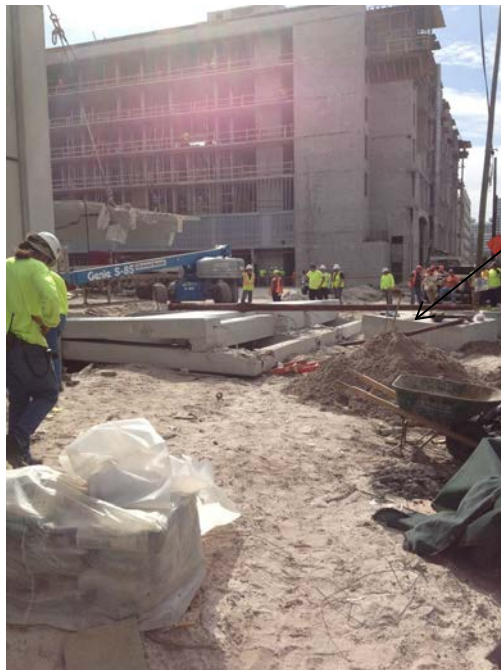
Fig. 15 Deadmen offset to pipe braces and walls
