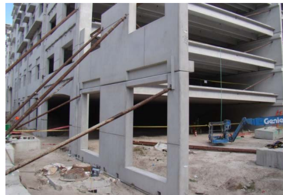
Fig. 35 Two Bracings per wall (post-incident)
