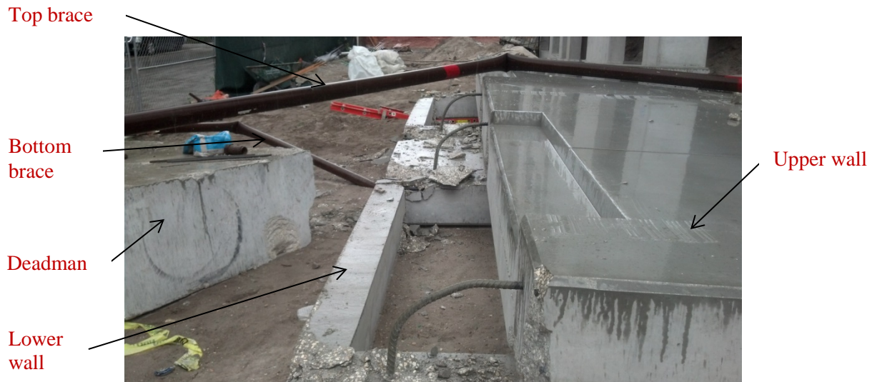
Fig. 10 Failed walls and deadman
