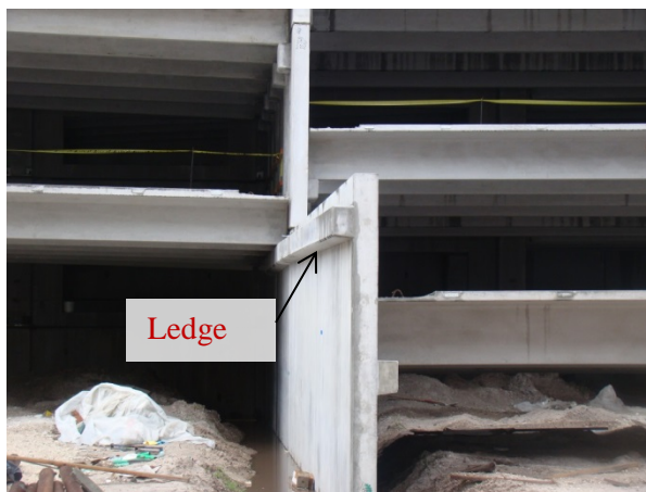
Fig. 22 Ledge on east side ramp wall (looking north)
