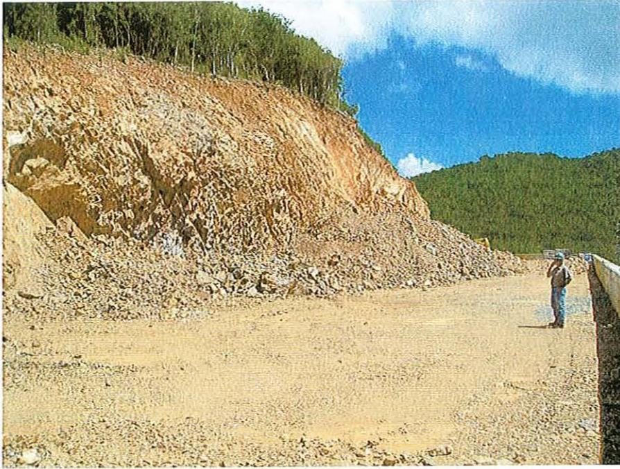
Figure 21. Identifiable Rock Slabs in the Excavation Face South of the Collapsed Area, Looking Toward Northwest.
