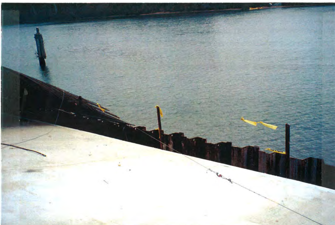
Figure 3-22 The Middle Portion of the South Guy Wire. Please note that there was no latch on the hook in this portion of the guy wire.
