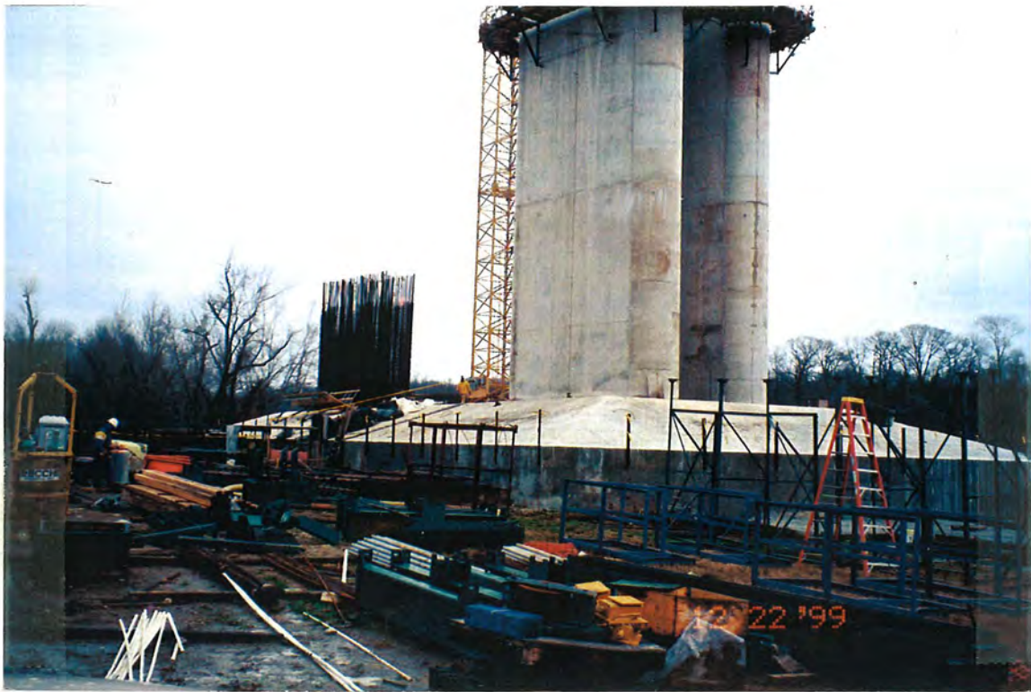
Figure 3-3 Site Condition around the Concrete Footing (Looking toward Northeast).
