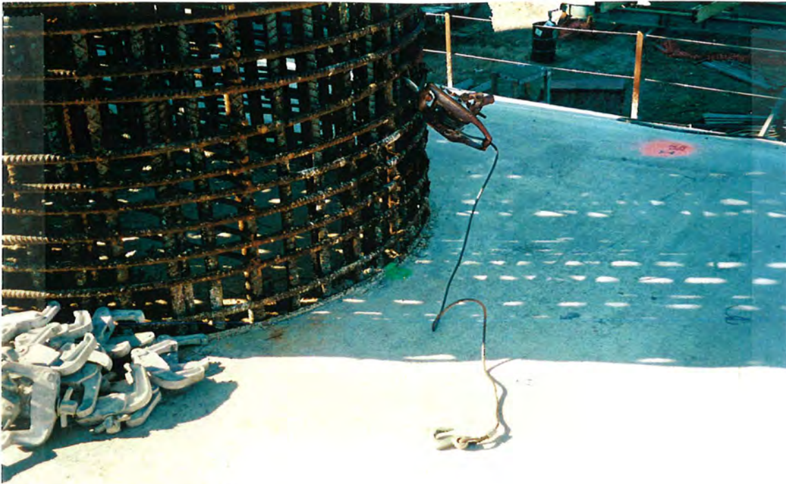
Figure 3-17 The Lower Connection Point of the Northwest Guy Wire at the North End of the Steel Cage for Column 1 of Bridge Pier WB-12.
