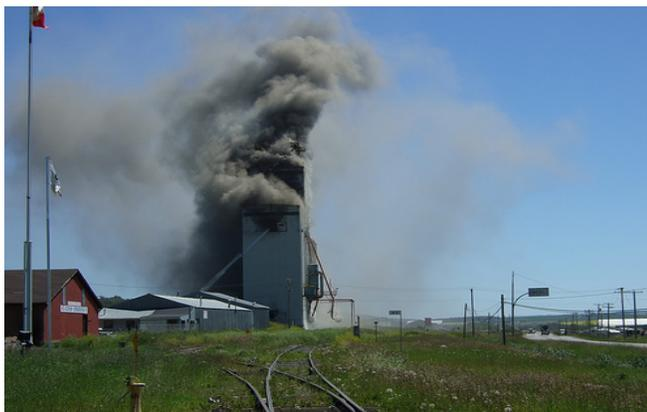
This causes a very rapid burning with a release of gaseous products and subsequent pressure rise. The resulting explosive force can damage plant, property, and people. Dust explosions can be categorized as either primary or secondary.
