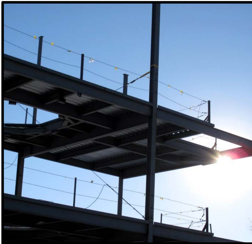
Wire Rope Guardrails with Flags
