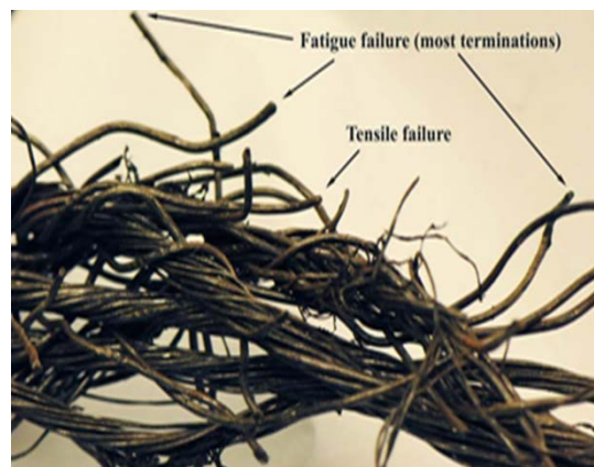
Photo 2: A portion of the failed wire rope section showing an excessive number of fatigue breaks in any length. Photo by: Daniel T. Crane, OSHA/DTSEM/SLTC
