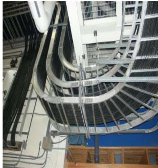
Figure 3. Electrical wires in multiple cable trays.
