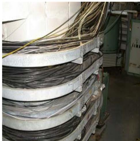
Figure 6. Overloaded Cable Tray.
