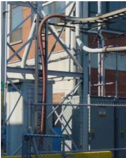
Figure 2. Outdoor metal clad cable in cable tray.
