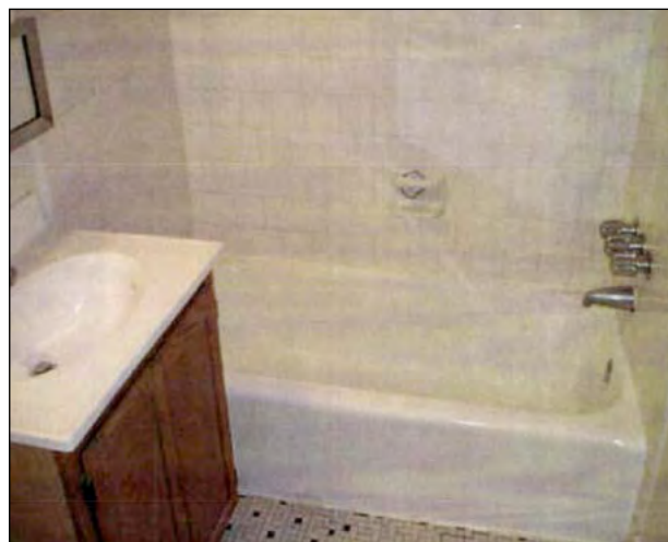
Photo courtesy of Maryland Occupational Safety and Health
