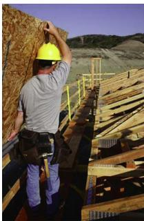
**Scaffolding:** Workers installing roof sheathing may be able to use scaffold systems. Bracket scaffolding systems, including top-plate scaffolding systems, can provide workers with stable work platforms. Workers may be able to install the bottom row of roof sheathing while they are standing on these scaffold systems and leaning over the
