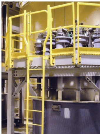
Raised platform with protected guardrail.
