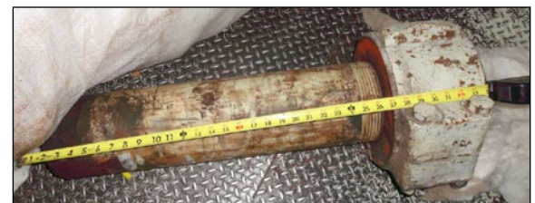
Figure 2: Portion of column separated from the main column in the incident. It is about 34 inches long and 7 inches in diameter.
