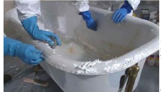
Workers use a methylene chloride-based stripper to remove paint from a bathtub prior to refinishing.
