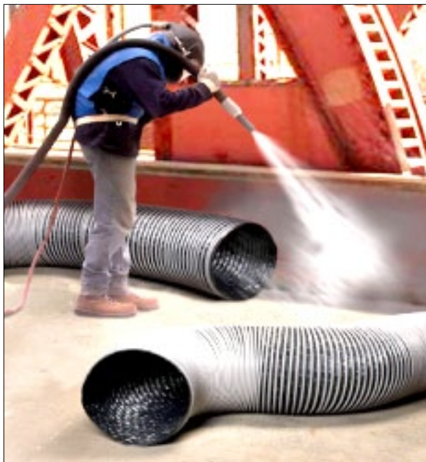
Abrasive blasting using a dust collection system with multiple exhaust ducts. (Photo courtesy of Flexaust, Inc. This equipment is shown for illustrative purposes only and is not intended as an endorsement by OSHA of this company, its products or services.)
