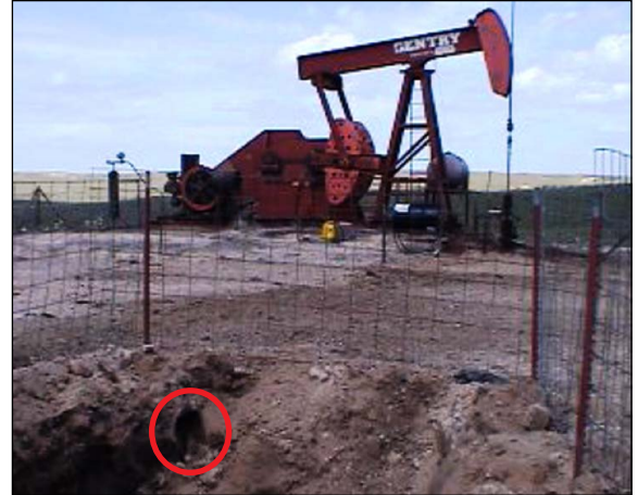
Cut end of pipe in trench.
