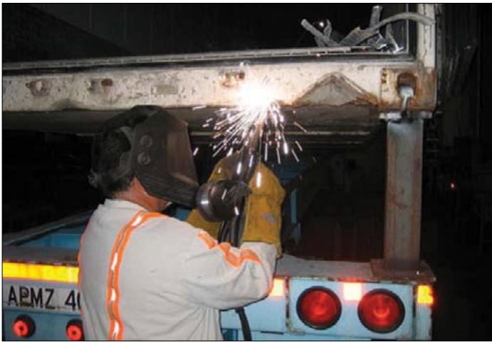
Figure 2: Welding the rear sill of a container.
